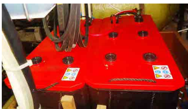
24V Engine Start Batteries
