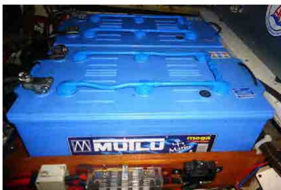
24V System House Batteries
