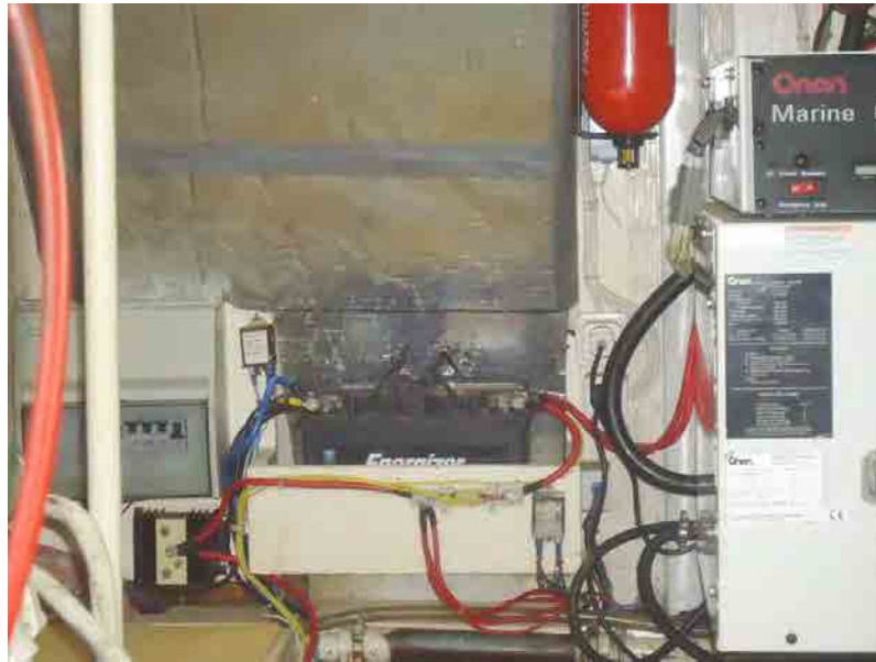
12V Breakers – 12V Battery(new), Onan 7Kv generator. Note automatic fire extinguisher.
